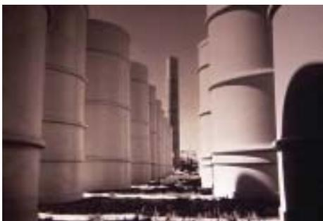
FRP has been used extensively in chimney liners exposed to sulfur dioxide and sulfur trioxide. Wet scrubbers and ancillary equipment associated with flue gas desulfurization processes can represent extremely corrosive environments to carbon and stainless steels, whereas FRP is quite resistive.
