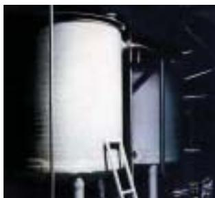
Carbon steel, stainless steel, rubber-lined steel, and premium alloys, once standard materials of construction for chemical storage tanks, are more and more being replaced by fiber reinforced plastics (FRP) as engineers begin to realize the advantages of FRP, e.g. increased corrosion resistance, light weight, higher strength to weight ratio, low life cycle costs, etc.
