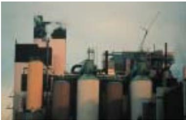
FRP has long been a material of construction for pulp washer drums used to extract residual chlorine dioxide or caustic chemical carryover from pulp. FRP is also used in large diameter up-flow tubes and retention towers where digested wood chips are first chlorinated and then bleached in the pulping process.
