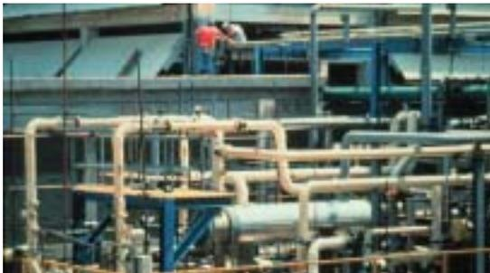
FRP piping is used extensively in process piping systems, stock and effluent piping in pulp bleach plants, chemical waste and municipal waste sewer piping, cooling tower piping, leach field acid piping, irrigation piping, etc.
